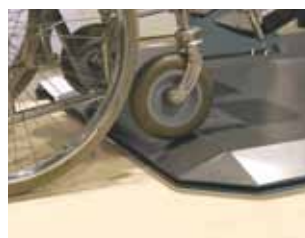
Fixed inclined edge for connection with lower landing
